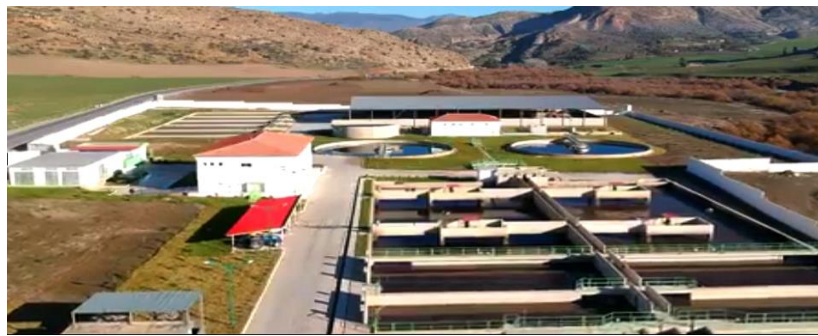
Figure 1 : Station d'épuration Ain Baida Harriche (ONA 2018).
